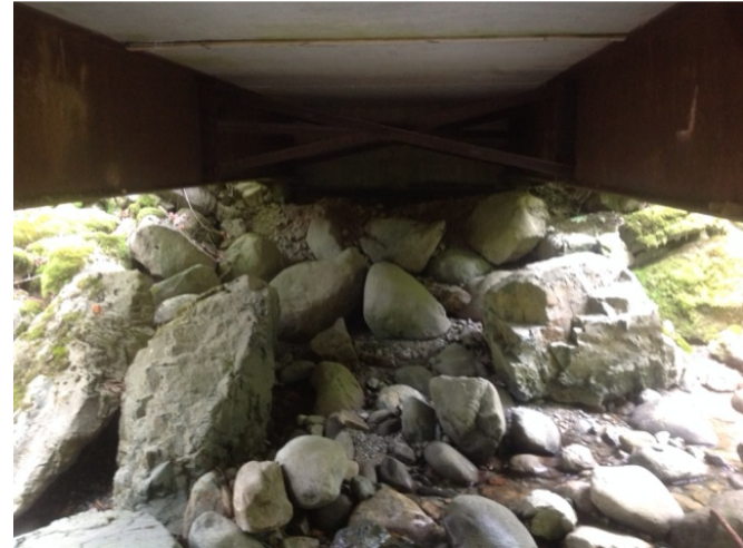
Right Bank Abutment when facing downstream
