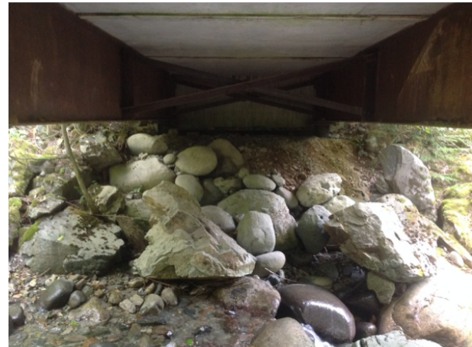
Left Bank Abutment when facing downstream
